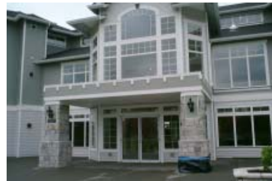
entrance with portico and ornamental treatments
