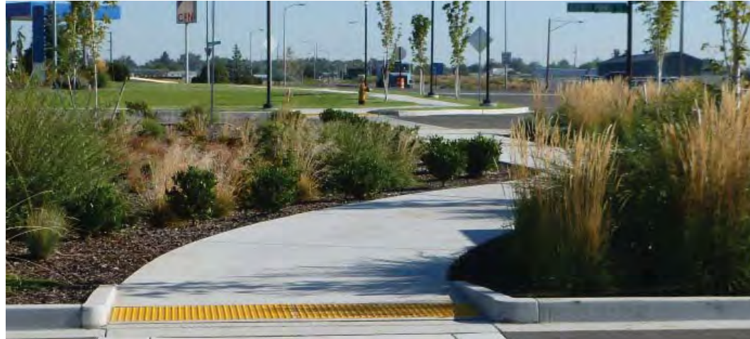
Sustainable landscaping used to accentuate trail/walk crossings through parking lot.
